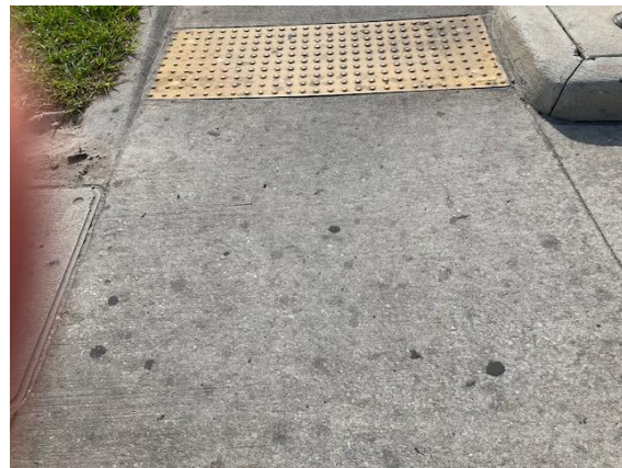
5.11.26 Sidewalk area without the solvent pressure wash
