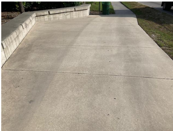
5.11.26 Sidewalk pressure washed with solvent
